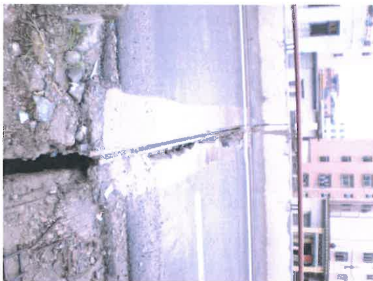
伸缩缝破损
