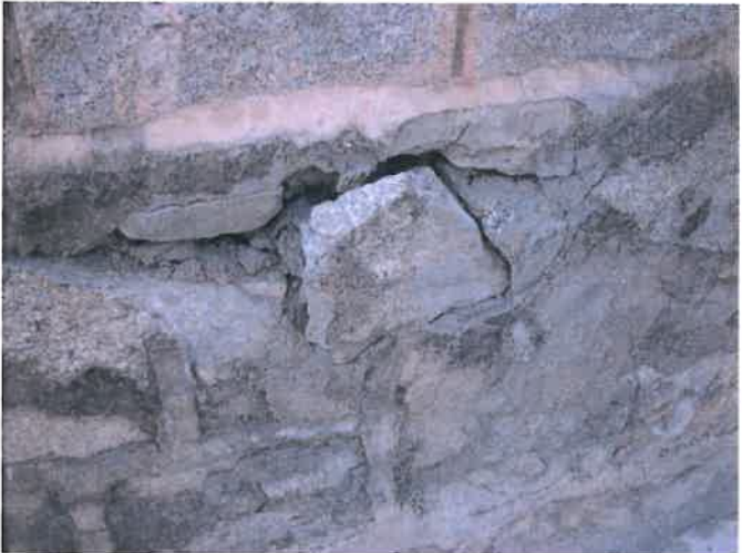
挡土墙破损
